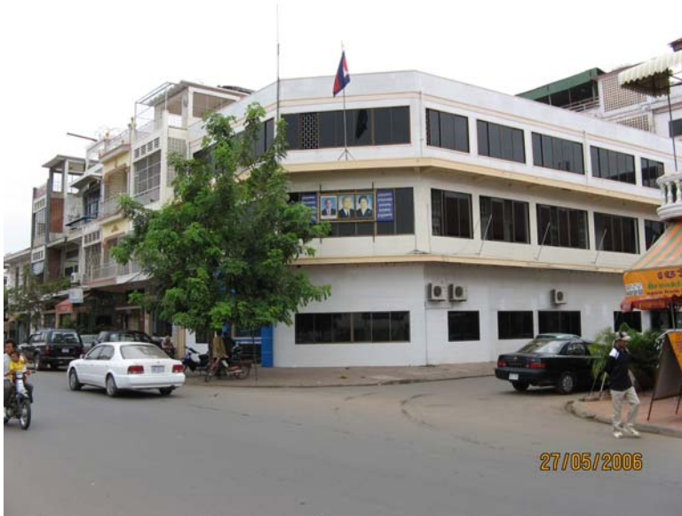
Kam Sab Office Upgrading Project Preah Sisovath Quay, Phnom Penh Owner: Kampuchea Shipping Agency & Brokers (KAMSAB)
