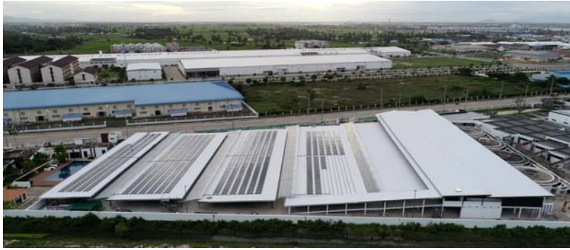
Laurelton Diamond Extension Project P02- Locker Room, Motor Bike Parking and Cover Walkway at PPSEZ Phnom Penh Client: Laurelton Diamonds (Cambodia) Co., Ltd. Consultant: Archetype Cambodia
